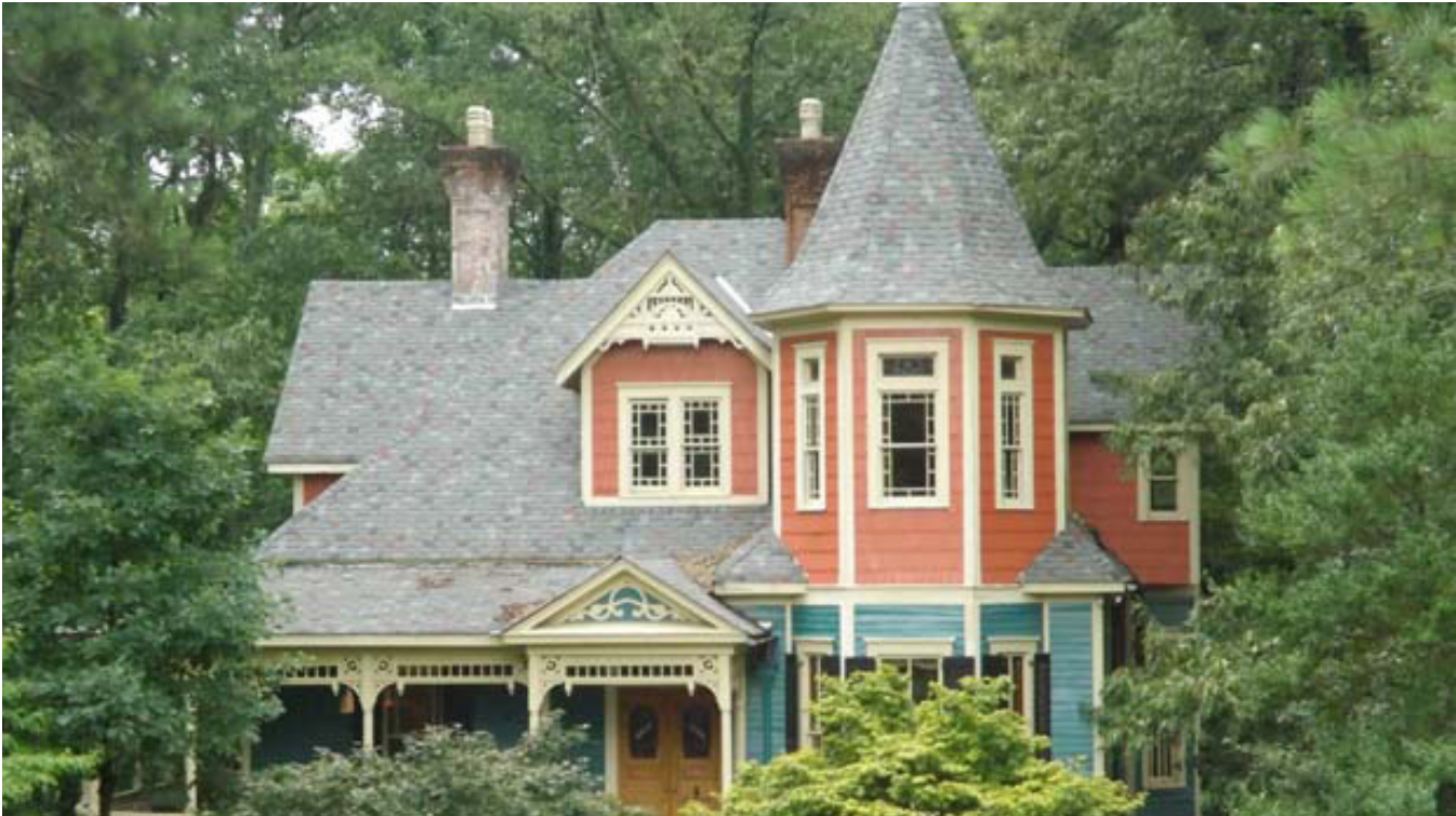
Figure 4. Example of Contemporary Structure with Historic Detailing
