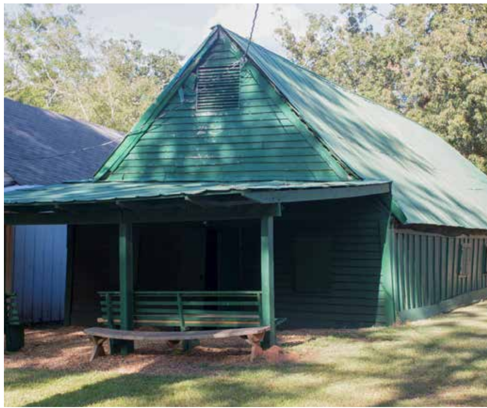
The earliest tent (c. 1840), Cunningham-Ramsey , began the trend of rectangular, front gable structures with large front porches and entrances on the short ends. A notable feature is the use of wood shavings as ground cover in both interior and exterior spaces.
