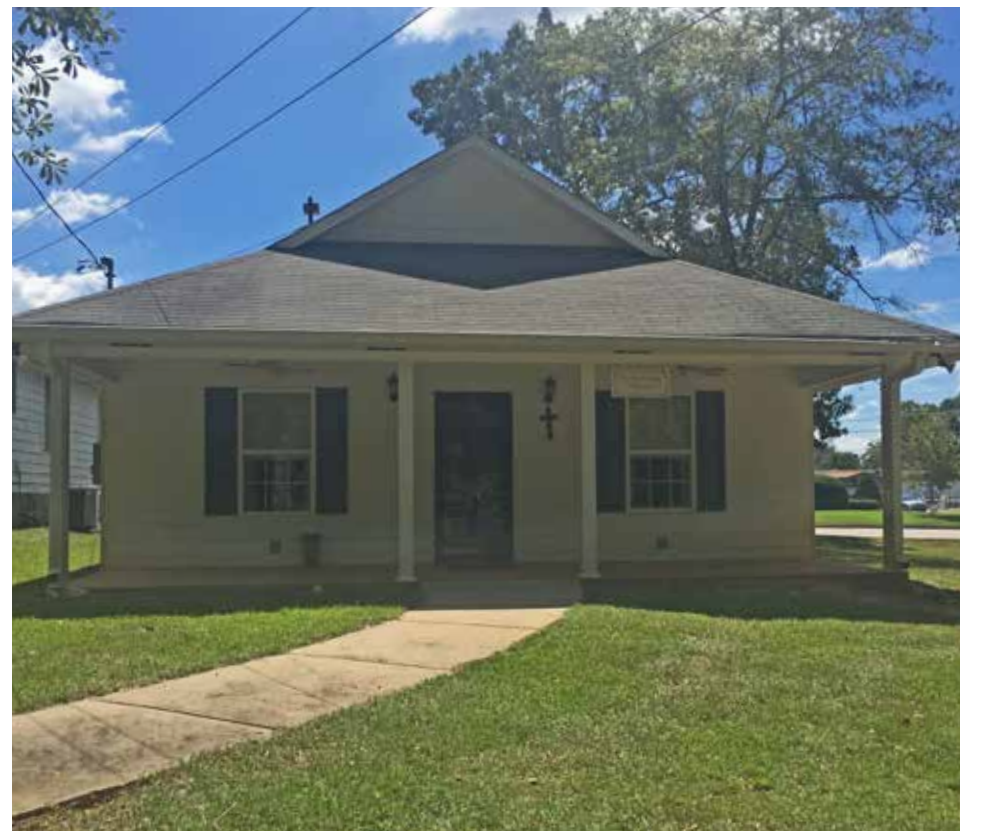
Piper-Head serves as an example of a contemporary tent, built in 2010. The tent maintains the traditional configuration while using new materials like vinyl siding, mimicking the wooden clapboard used historically.
