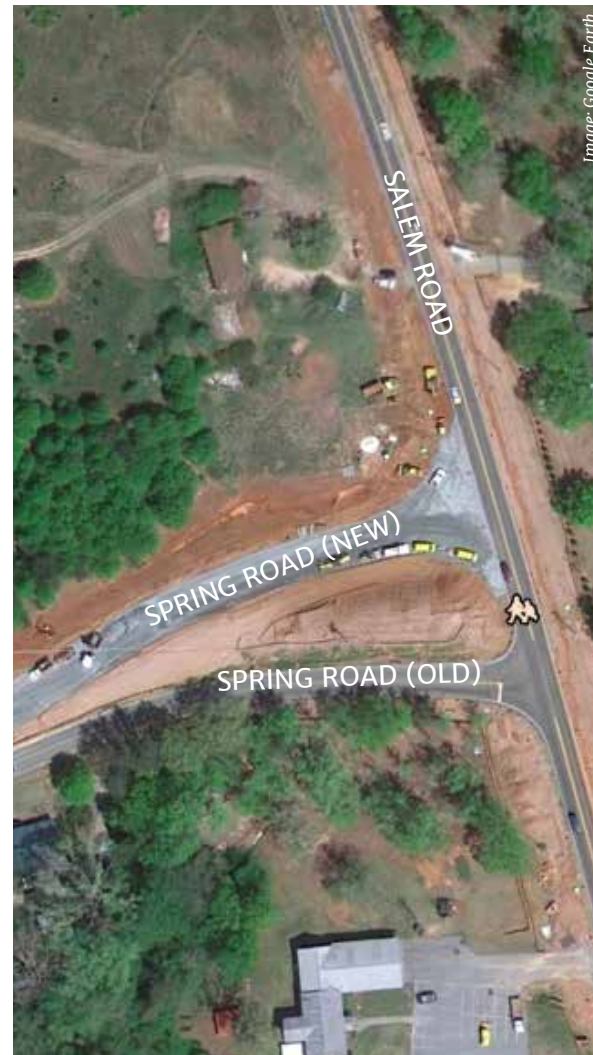
2010 Spring Road relocation project
