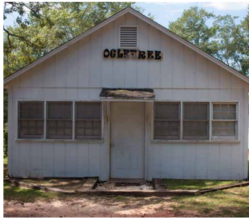
Ogletree is an example of a tent that has received several material changes over the years, while maintaining its overall design. Rather than wooden clapboard, it is clad in a more contemporary composite vertical board siding. The porch ground cover has been updated to paving. Sash windows are present but in a similar layout as on the Cunningham-Ramsey tent.
