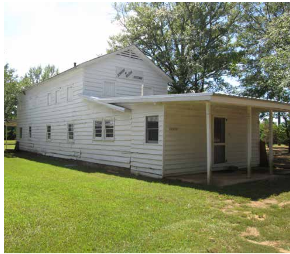
Jenkins-Milton serves as an early example of a two-story tent within Salem Camp Ground. It maintains the same general configuration as the one-story tents, but with a second story. There are only three other two-story tents present on site.
