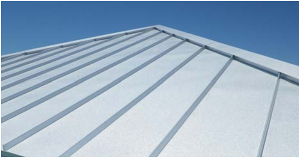
Figure 4.2: Architectural Guideline - Silver Standing Seam
