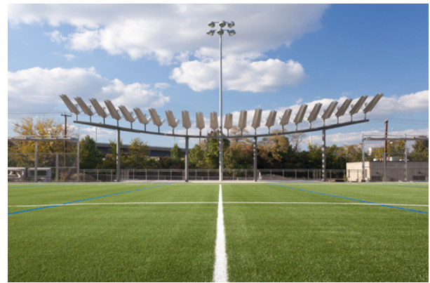
Figure B.11: Arbor at Long Bridge Park
