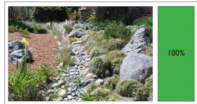
Stormwater Solutions: Dry Creekbed
