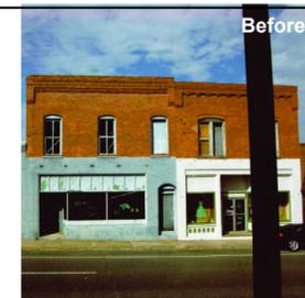
This brick on this commercial building needs to be inspected and repaired or repointed as needed. Boarded up windows in the second story should be returned to windows to maintain the rhythm of space to voids. The storefront is original to the building and therefore should be preserved and maintained. If cleaning and/or stripping is to be performed, use a gentle water-based or chemical treatment, never sandblasting.
