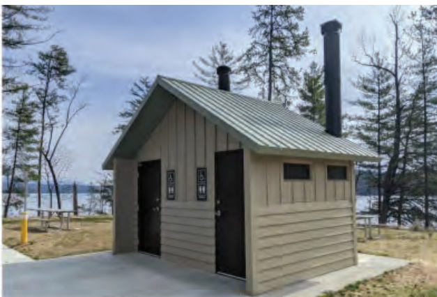
Prefabricated Pit Toilet
