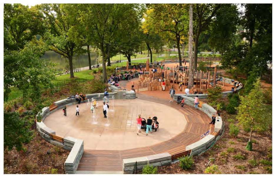
110 th Street Playground uses benches and seat walls to border the play area which keeps parents engaged and creates a nice physical barrier to the outside.
