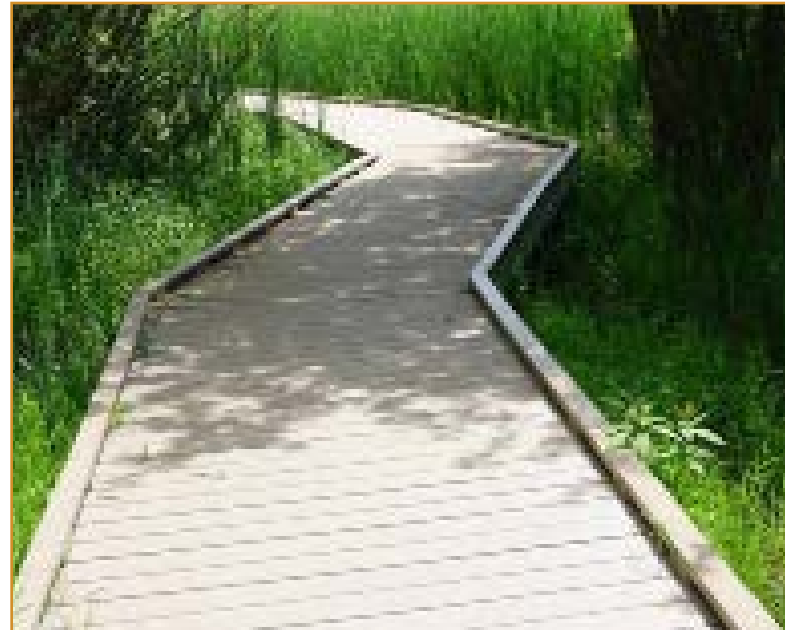
PRE-CAST CONCRETE BOARDWALK
