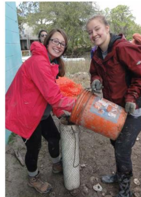
Landscape Architecture students bag oyster shells for the living shoreline stabilization project at the Burton 4-H center on Tybee.
