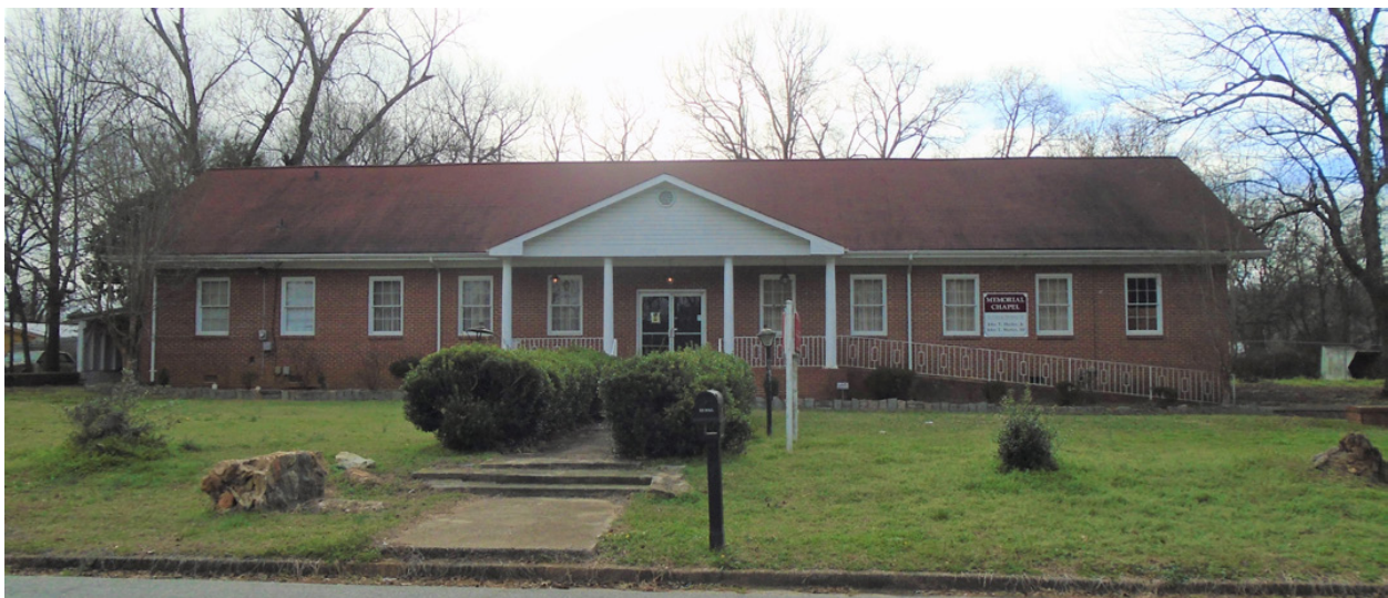
Figure 4 – The former Newtown Grammar School, which has been converted into a funeral home
