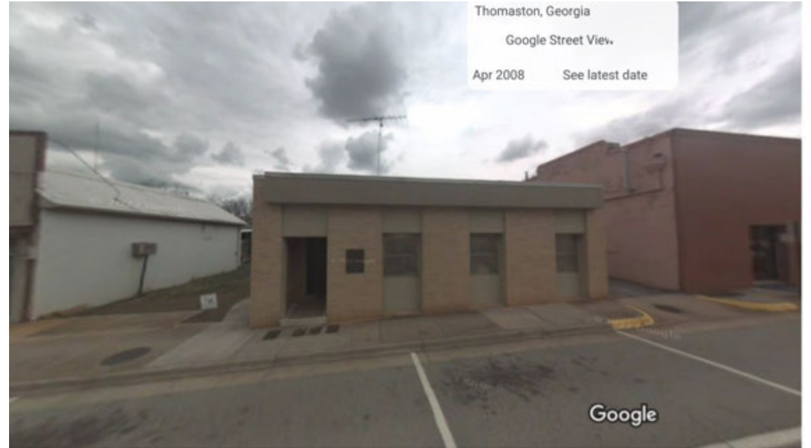
2008 Streetview showing façade. The building appears to have been renovated c. 1979, historic photos prior to that (ideally 1950s) would be beneficial to determine appropriate façade treatment options.
