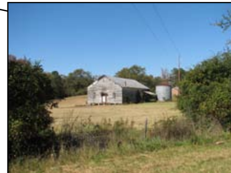
Barn with silo in field adds to the rural vernacular.
