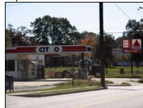
Abandoned gas station falling into disrepair
