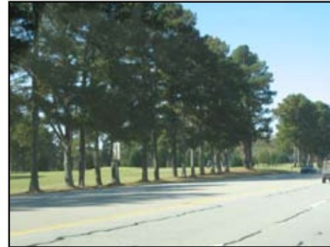
Transition into 4-lane road at Highway 80 Intersection.
