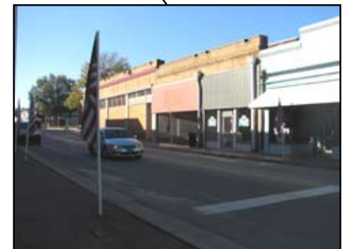
PVC pipes cheapen the aesthetic of downtown Washington
