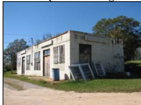
Abandoned building to be restored.
