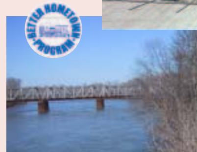
The existing steel truss railroad bridge inspired the design of the gateways signs. Primary entrances are inspired by the frontal view of the bridge, while the secondary entrances are inspired by the side view of the bridge. All gateway signs should be constructed of steel.
