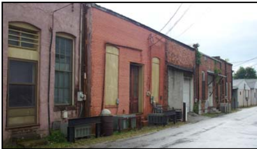
The HVAC systems create clutter. By cleaning up the backside of the buildings, Sandersville's downtown will expand by at least a block. Visitors and residents will be able to use the parking lot and feel safer as they walk through Jernigan St.
