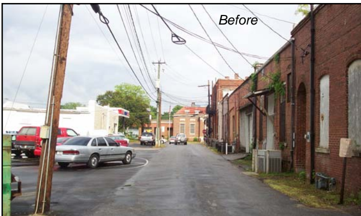
Existing leaning pole and power lines on Jernigan Street.
