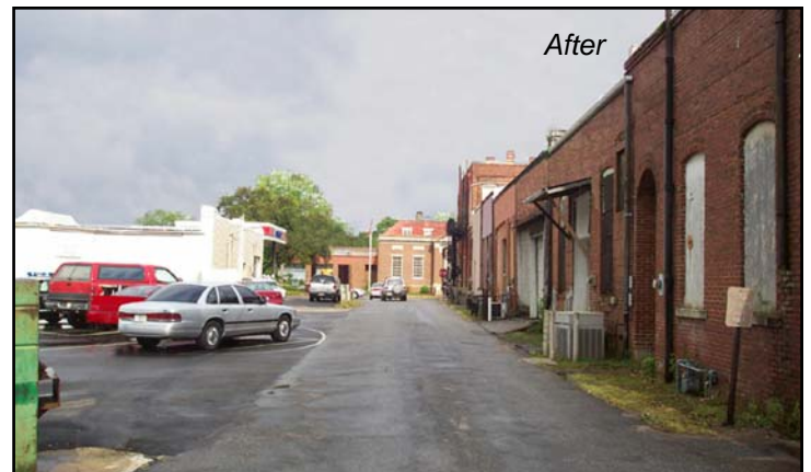
Visual clutter is minimized by burying the lines underground
