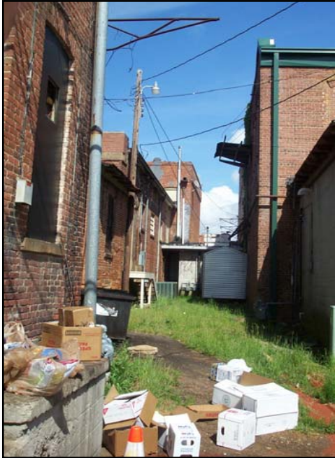
View of alley -- existing conditions
