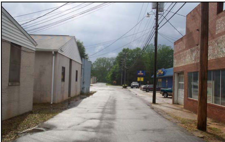
Jernigan Street has no sidewalk and is visually cluttered by power lines.
