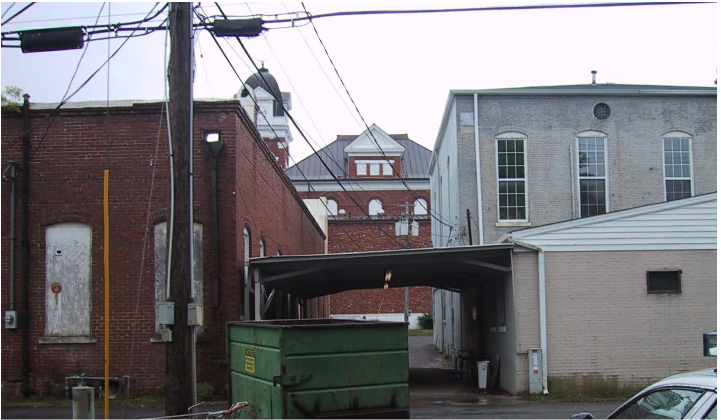
This alley appears run down due to the dumpster, boarded windows, cracked pavement, and looming power lines.
