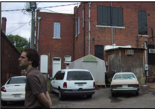
Boarded up windows and hap-hazard parking
