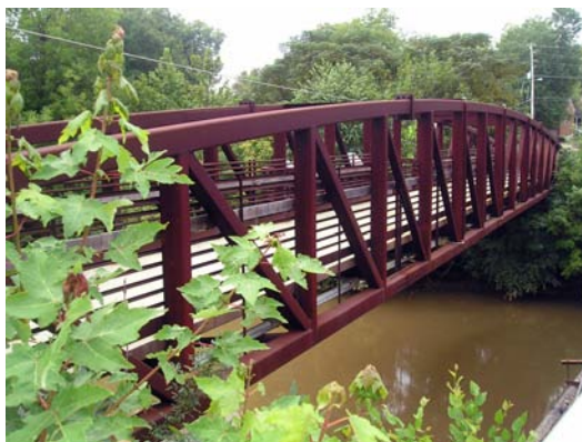
Example of a weathered steel bridge on a recreation trail
