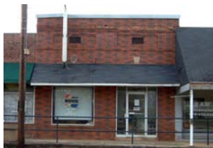
Historic elements obscure through improper renovation.
