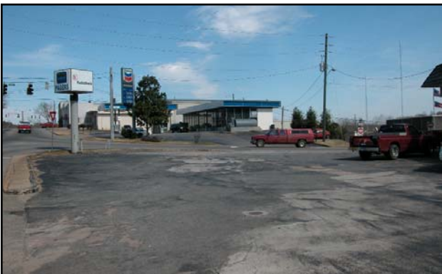
No markings on a vast expanse of asphalt makes for inefficient parking.
