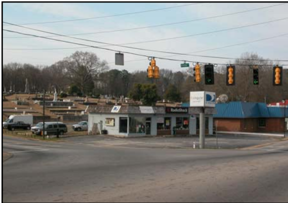
This corner can be redeveloped to create a grand park-like entrance to Woodbine Cemetery, or with a more attractive building for the existing businesses.
