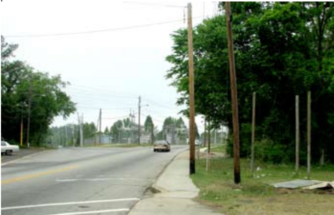
This sidewalk is too close to vehicular traffic to garner a feeling of safety for the pedestrian. Street - sidewalk separation should be at least 10' along Experiment Street.
