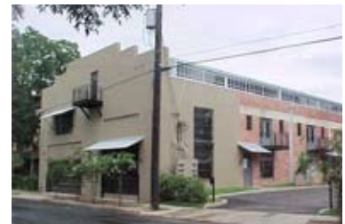
Existing building that many may think as eyesores should first be evaluated as potential buildings to re-use. This rather simple warehouse was rehabilitated using historic preservation tax credits and became a very popular place to live.
