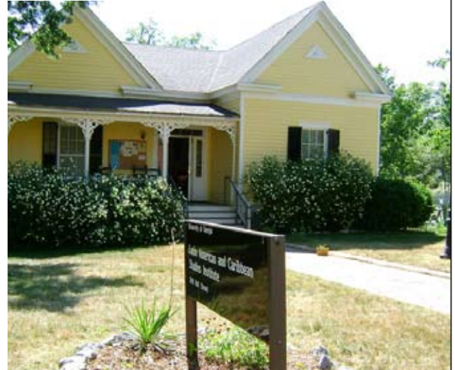
Similar structure surrounding many major Universities have been creatively converted to new uses as much needed administration offices.
