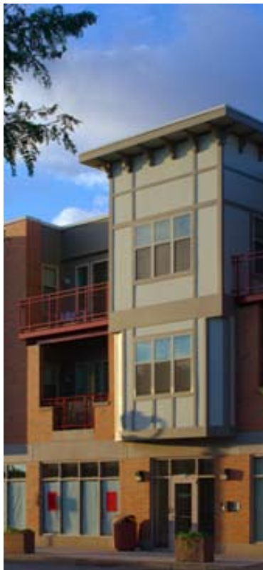
A multi-use affordable housing unit has retail on the street level with living above. It incorporates many of the elements discussed in this document yet is very contemporary and still handsome and compatible.
