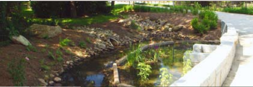
This raingarden was recently constructed during the Lumpkin Street Drainage Project.
