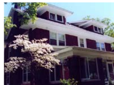
The ubiquitous “stacked duplex is a familiar sight across the nation. It still provides a good form for new housing along busy corridors.
