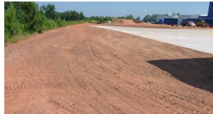
▲ Runoff near the building drains into a bioswale which connects to the upland bioretention pond to the existing detention pond for the industrial park.
