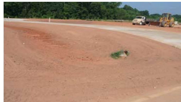
▲ The employee parking lot retention pond will accommodate a moderate rainfall event of 1-2".
