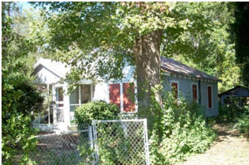
Photo 2: Custom-fit plywood that has been painted a festive color is a simple way to make a temporarily vacant home look worthy of living in by a prospective new owner.
