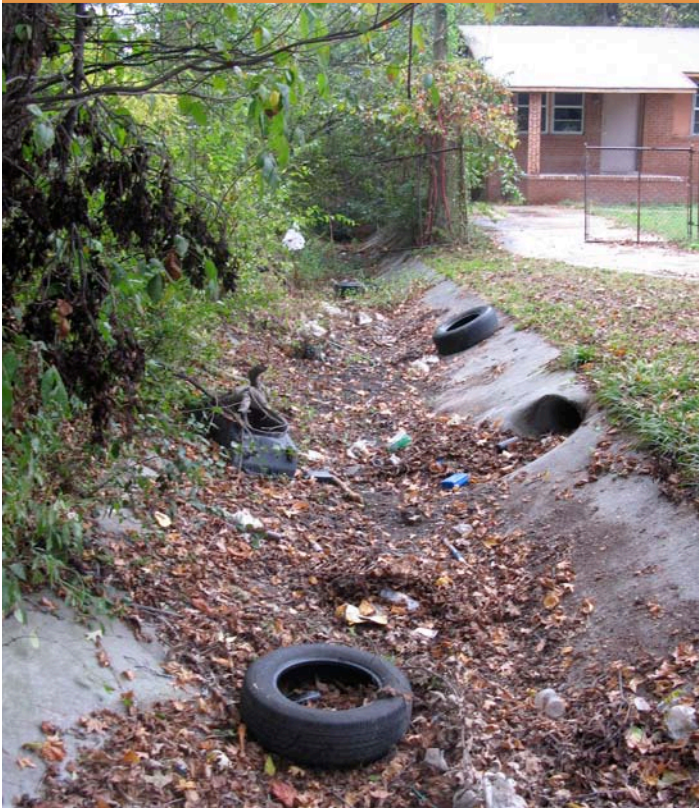
Besides looking unsightly, trash and tree debris inhibit the flow of water and promotes mosquitos. Regular maintenance in Hyde Park is necessary for free stormwater flows.
