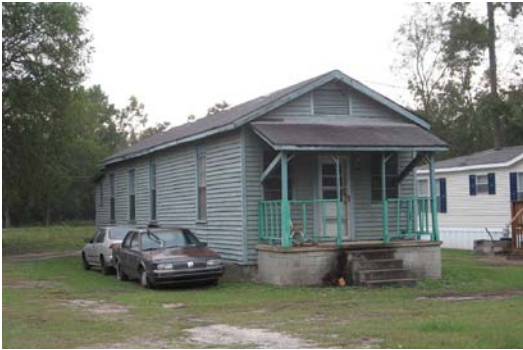
We found several great historic house styles, like the shot gun, bungalow and front gable-el, that are being used today as infill prototypes to solve the Gulf Coast Crisis.
