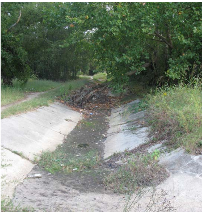
Besides looking unsightly, trash and tree debris inhibit the flow of water and promotes mosquitos. Regular maintenance in Hyde Park is necessary for free stormwater flows.
