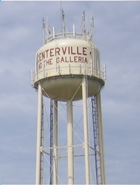
Centerville Water tower.
