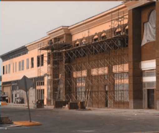
A two-story office building is created from the blank walls of a former department store in Chattanooga, Tennessee. (Courtesy of Dover Kohl & Partners).
