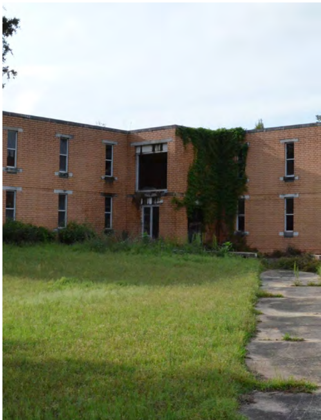
Nature is taking its toll on many of the campus buildings.
