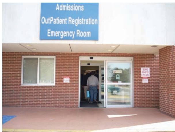
▲ SOME FEATURES OF THE HOSPITAL, HOWEVER, HAVE BECOME OUTDATED AND INEFFICIENT.
