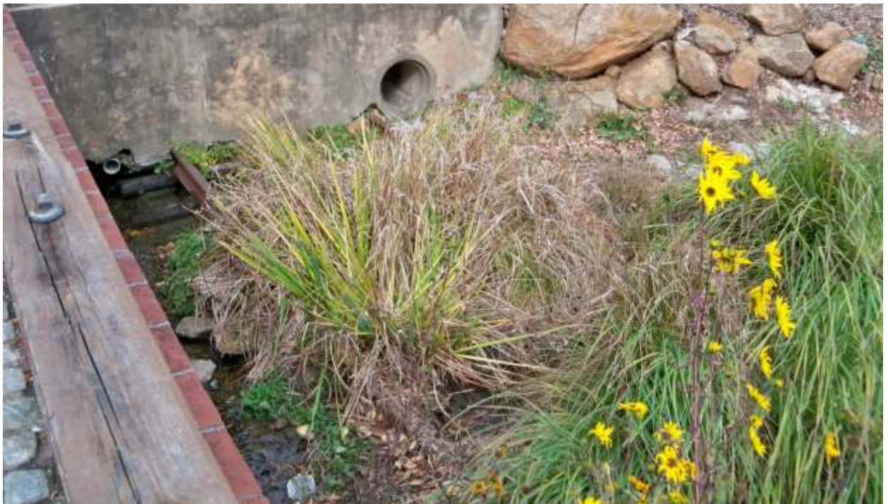
Figure 5: Restored section of spring with railroad tracks
