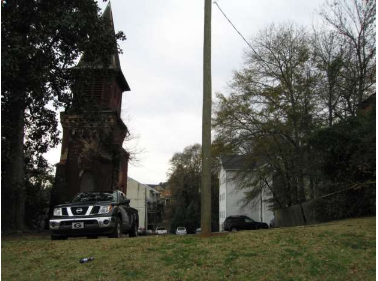
Figure 7: Saint Mary's Episcopal Church Steeple on Oconee Street
