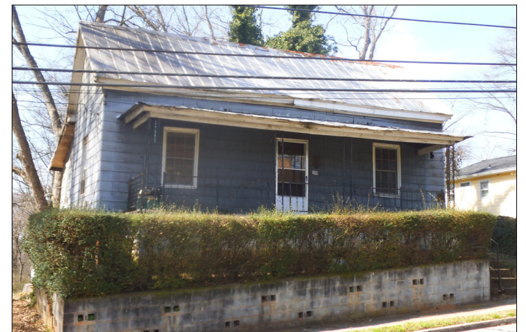
Porches, historic retaining walls, shallow setbacks and engaging yards give the neighborhood a unique physical identity.
