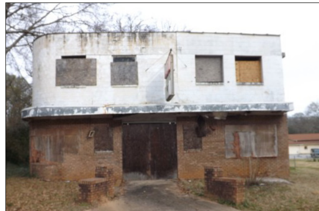
Existing American Legion Building condition
