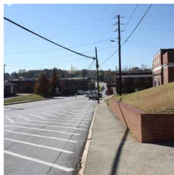
Additional parking spaces created by re-routing Cotton St. to intersect with Poplar St. and converting underutilized asphalt into parking.
