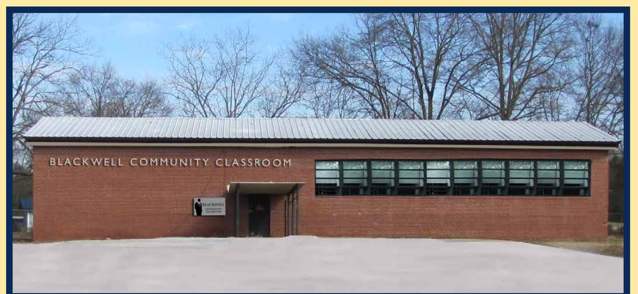
Repair windows and add signage
