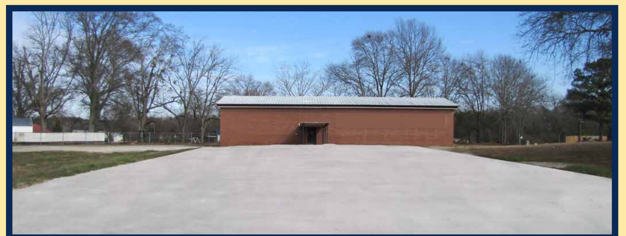
Skim-coat concrete and paint plywood
