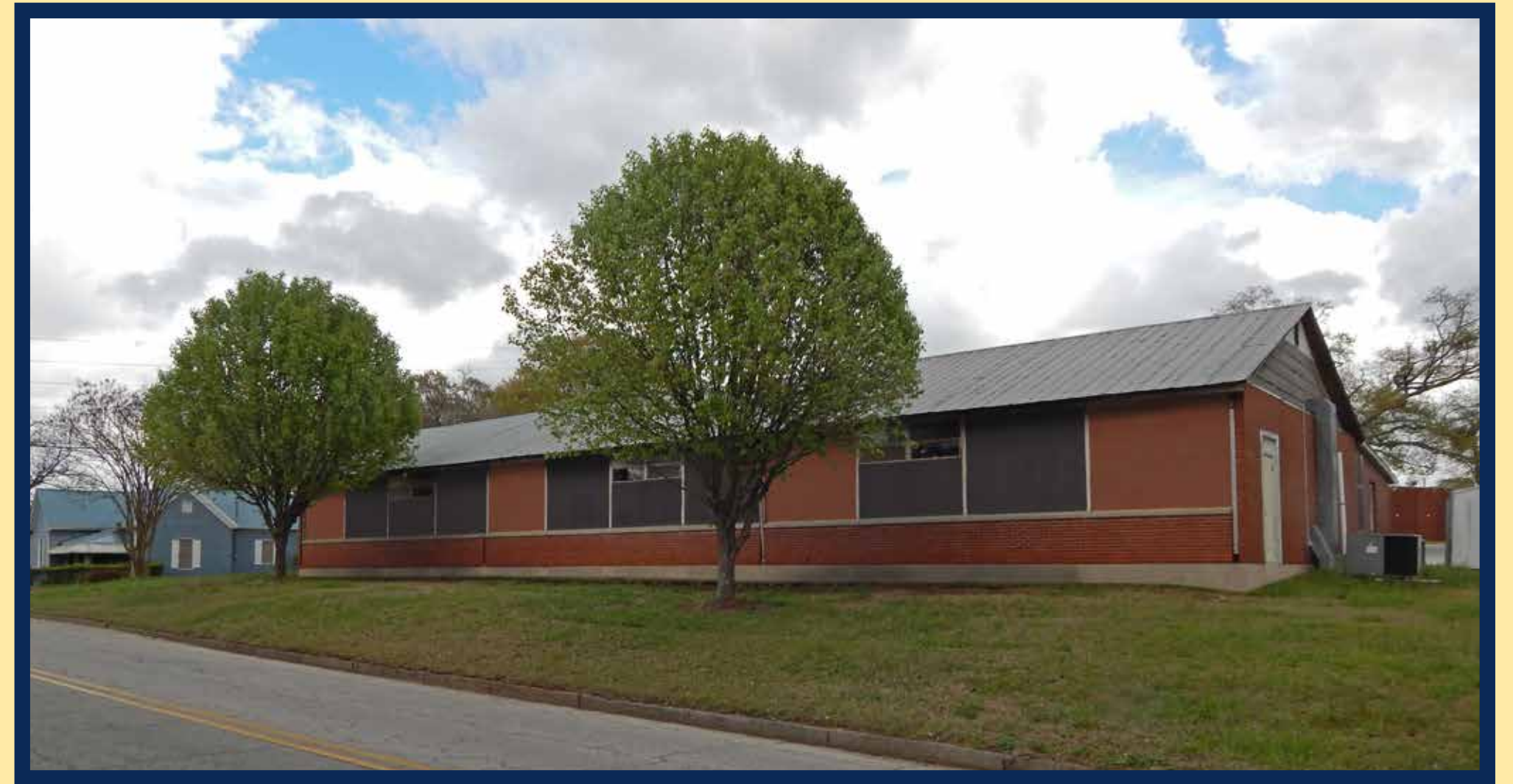
Paint cinderblock and plywood
