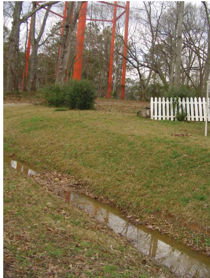
Swale draining overflow from water tower
