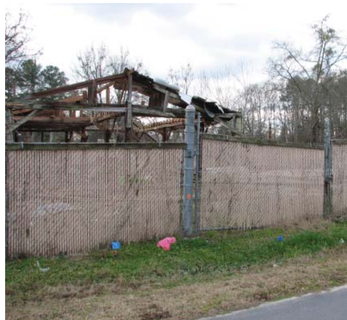
Maintenance shed area
