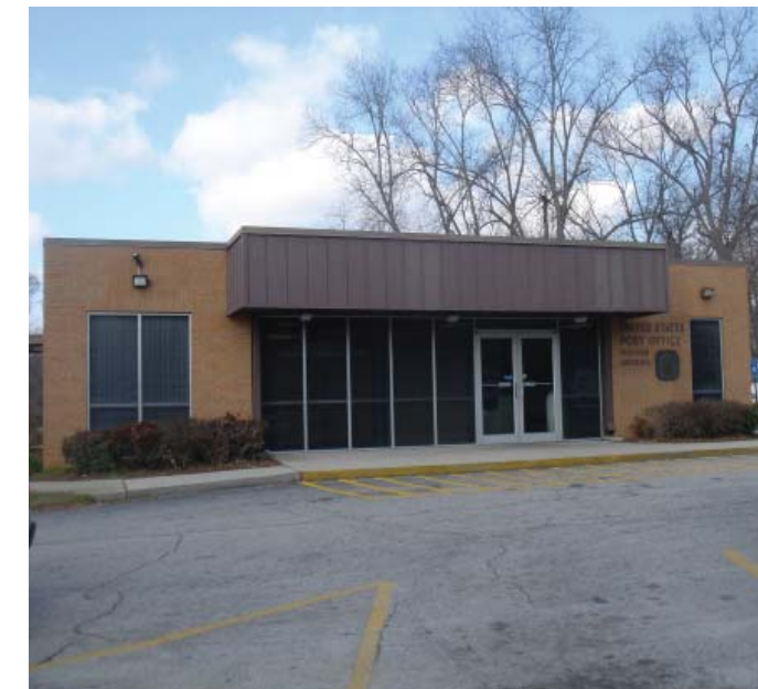
Post office function, but not building design
