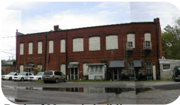
Back of Masonic building
