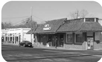
Existing conditions of Kay's Pharmacy
