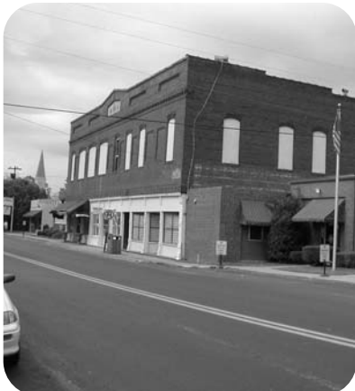
Existing conditions of Masonic building
