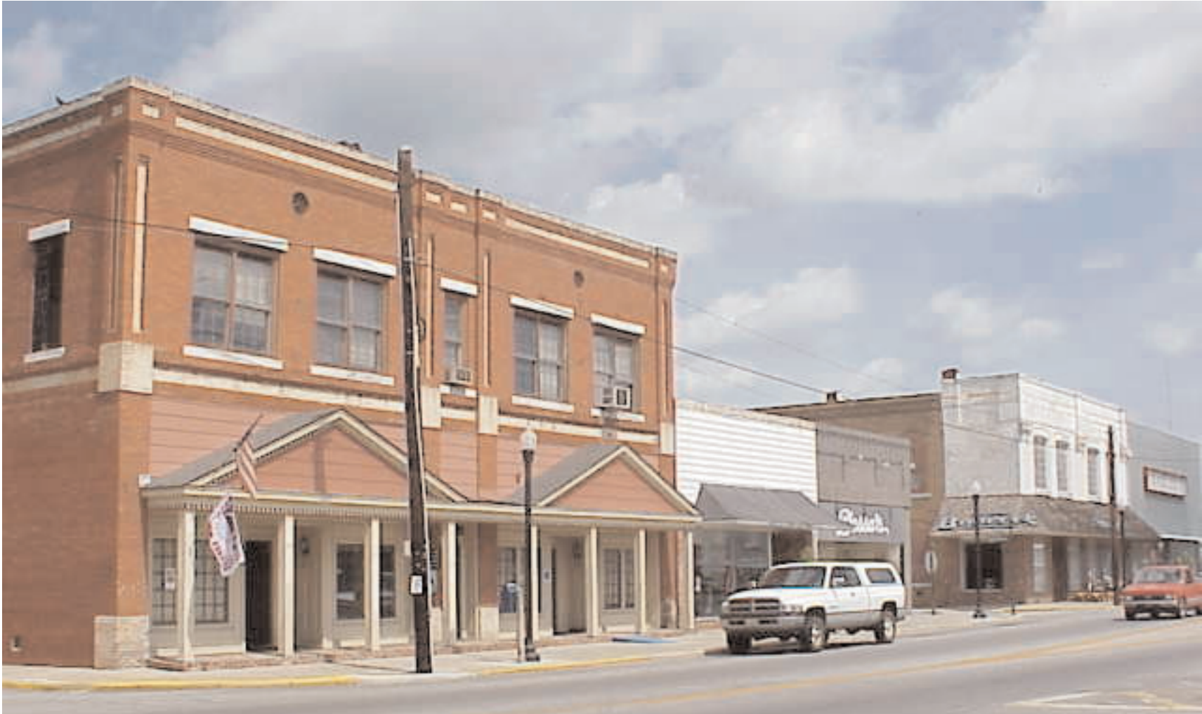
Existing Westside facades
