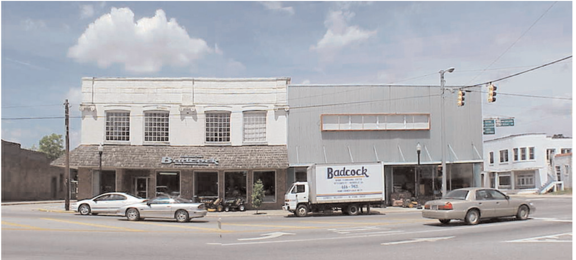
Existing Westside facades
