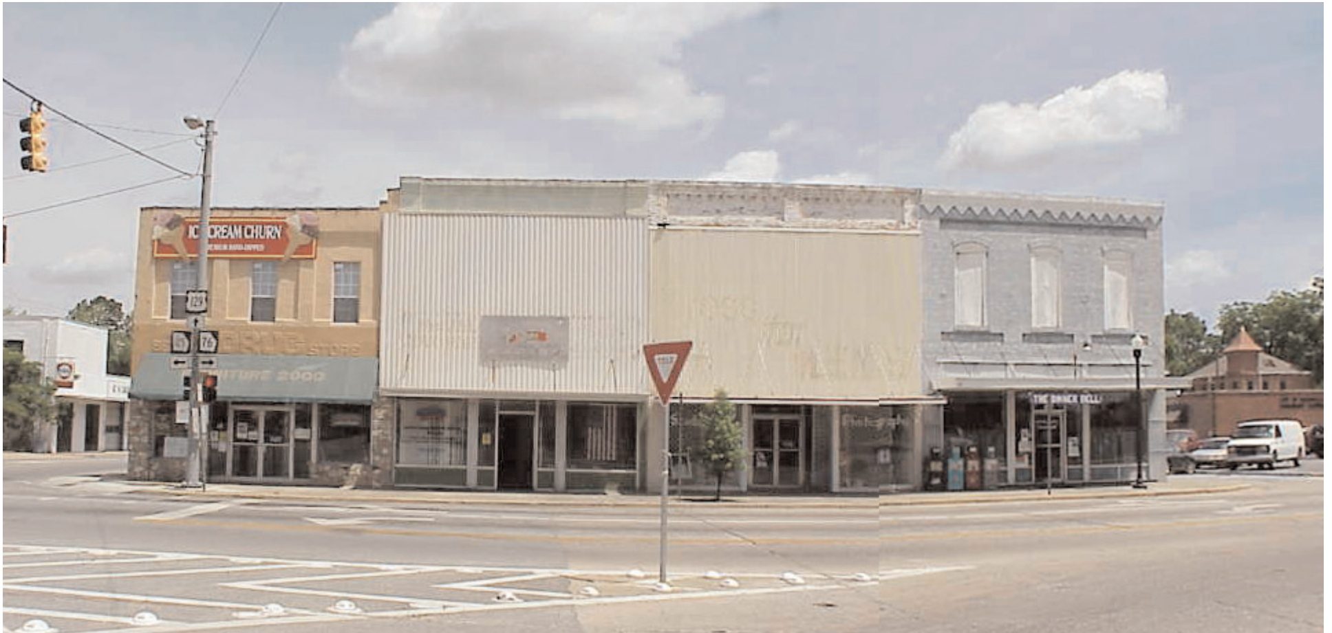
Existing Northside facades
