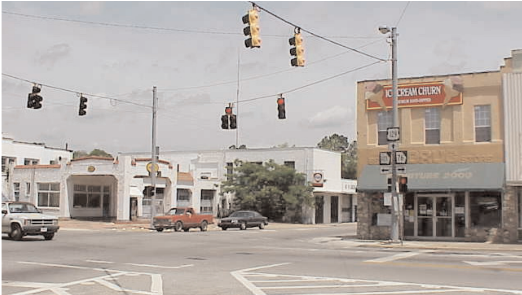
Existing intersection of Northwest corner
