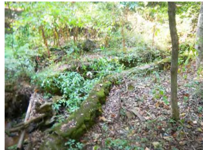
Spring and Walls Could be pre-1938. Concrete spring with two walls and a damn. Could have been used to water livestock or irrigate farmland. Area
