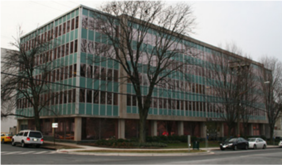
Figure 6. The American National Bank Building in Montgomery County, MD was designed in 1963 by architect Ted Englehardt. This building utilizes the brightly colored paneling that is typically found on large-scale midcentury modern architecture and also shows how architects would divide a building's facade into clear window bays through the use of aluminum molding
