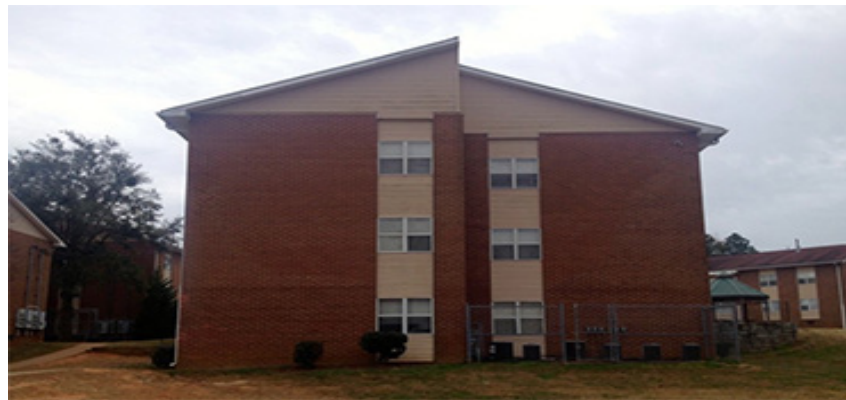
Figure 1. Photograph taken by Leeann Dickerson showcases the modernist roof line of Bethel's apartment buildings.
