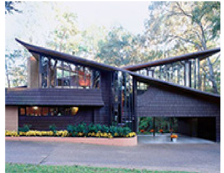
Figure 4. This home designed by architect Bruce Goff is an example of the butterfly roofline popular throughout the modernist architecture movement.
