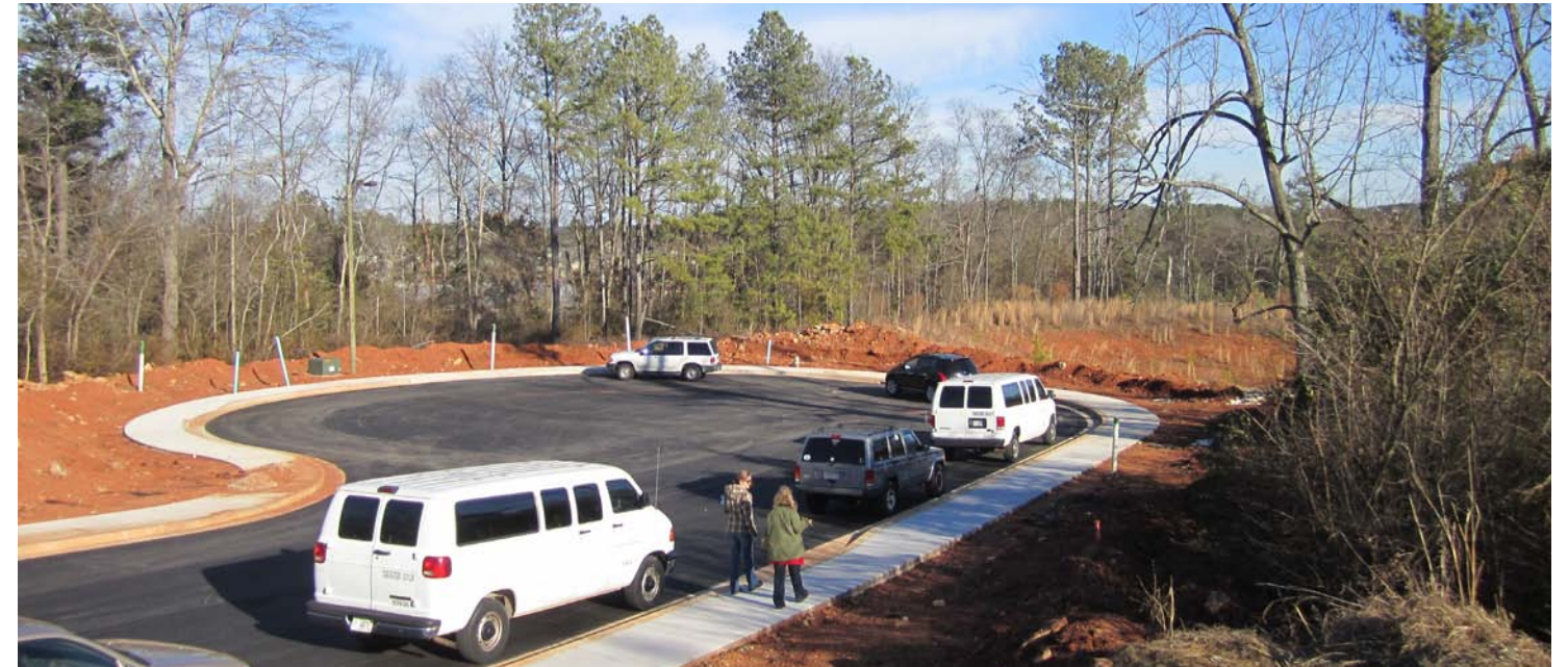
Figure 83 - The lack of human scale of the cul-de-sac is evident in this image in which the cars and individuals are dwarfed by the 96' diameter.
