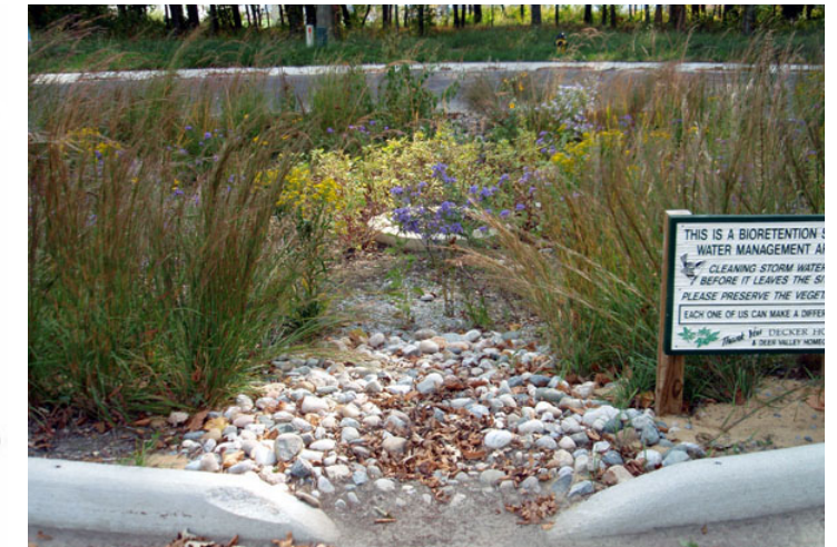
Figure 88 - This rain garden, located in Lucas County, Ohio, drains approximately 1.2 acres including driveways, front yards, and the roadway. Runoff is introduced through one of four curb cuts that are set equidistant around the perimeter of the rain garden.
