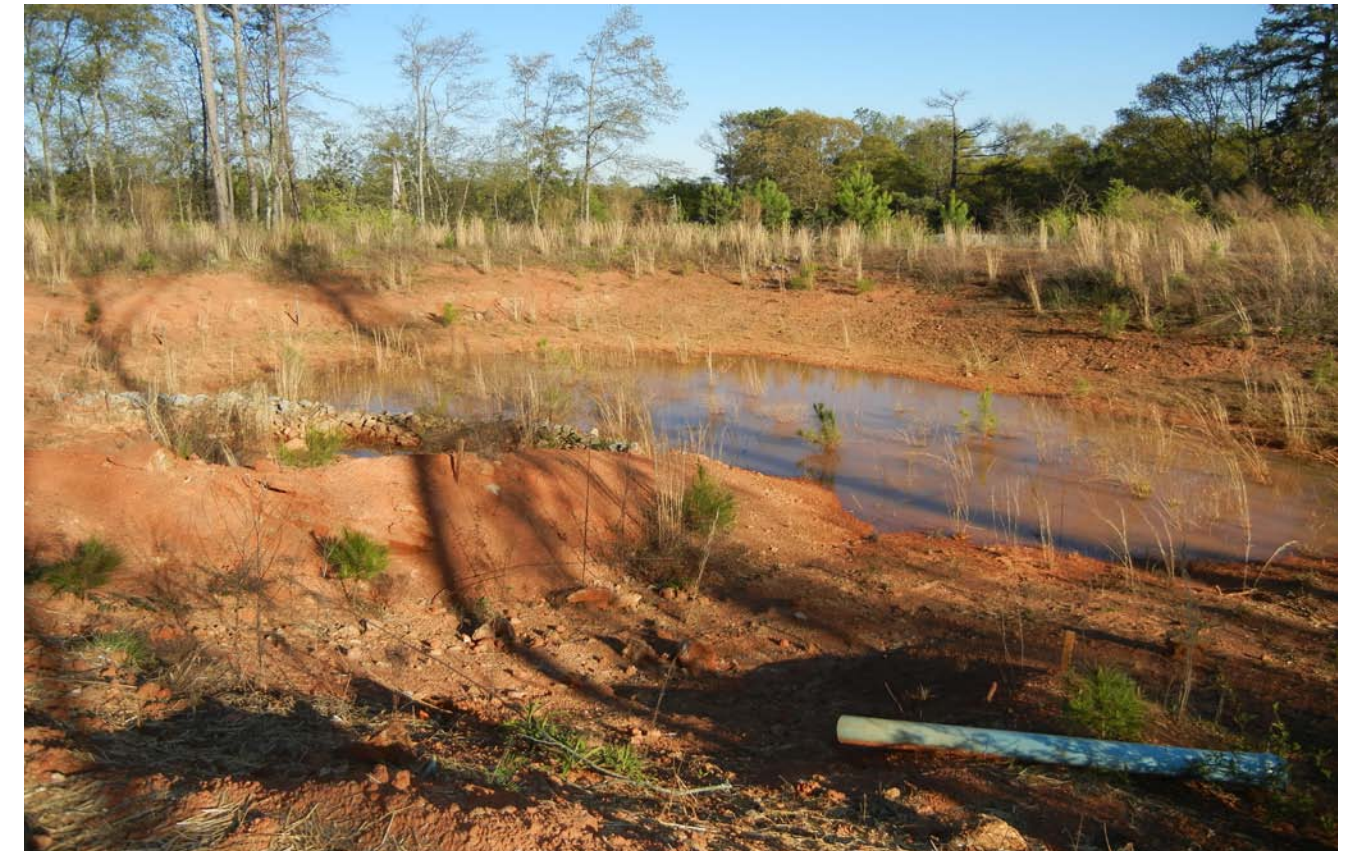
Figure 97 - Existing condition of the stormwater management area
