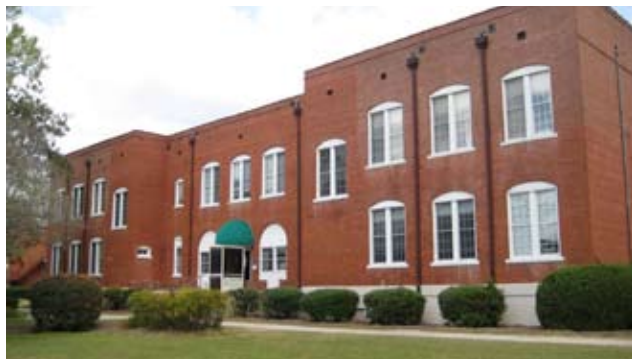
Existing: back of the building
