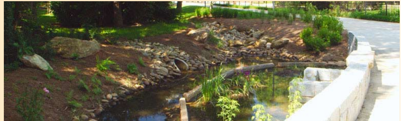
This raingarden was recently constructed during the Lumpkin Street Drainage Project.
