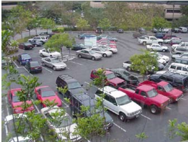
Parking lots can be curvilinear reducing the impervious footprint and interplanted with trees to help shade the space.
