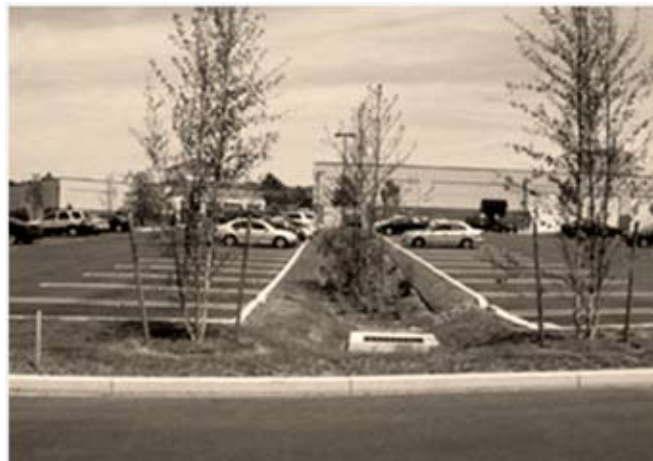
This parking lot is directing all the runoff into planted strips between the rows of parking. Appropriate plantings of Betula nigra , River Birch, were used because of their ability to withstand wet soils for an extended period of time.
