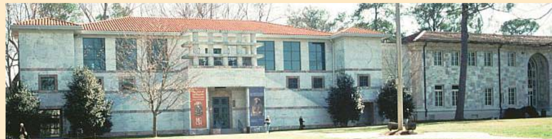
The law school building after the 1985 renovation
