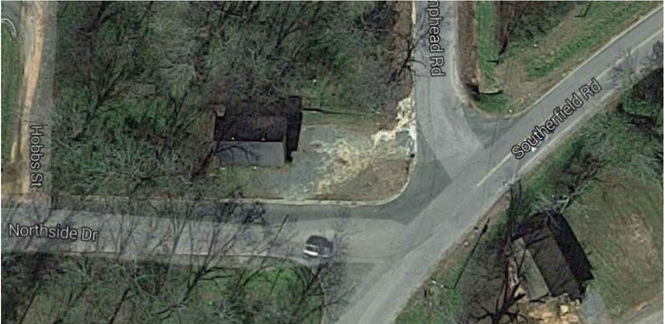
This five-way intersection at Bumphead Rd. is confusing and could benefit from a roundabout.
