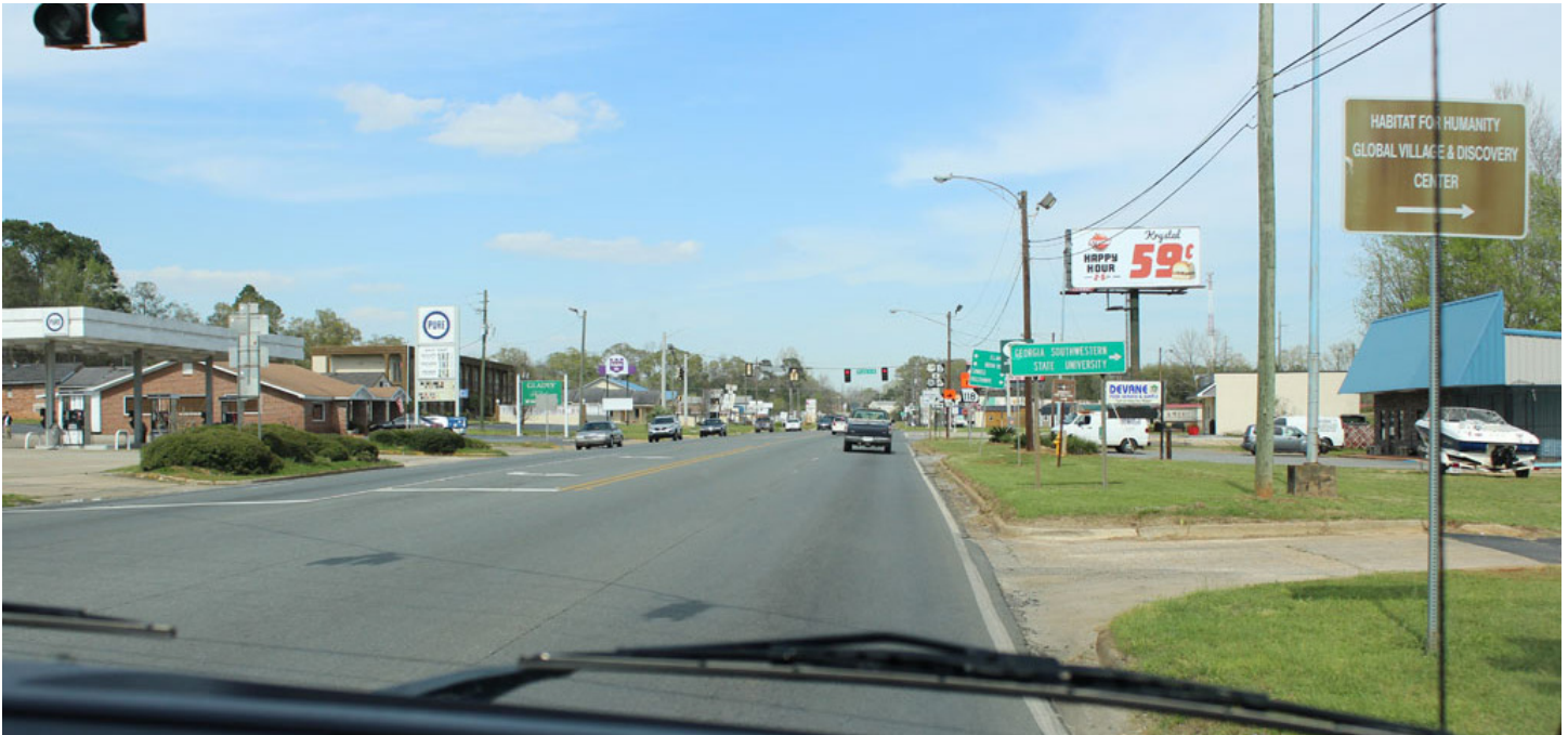
Existing conditions on Hwy. 19
