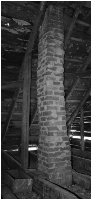
Figure 29: later chimney in attic
