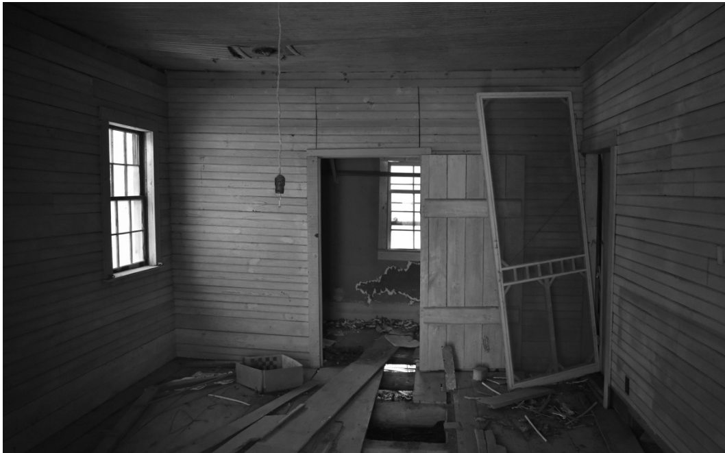
Figure 26: Room 104, looking south
