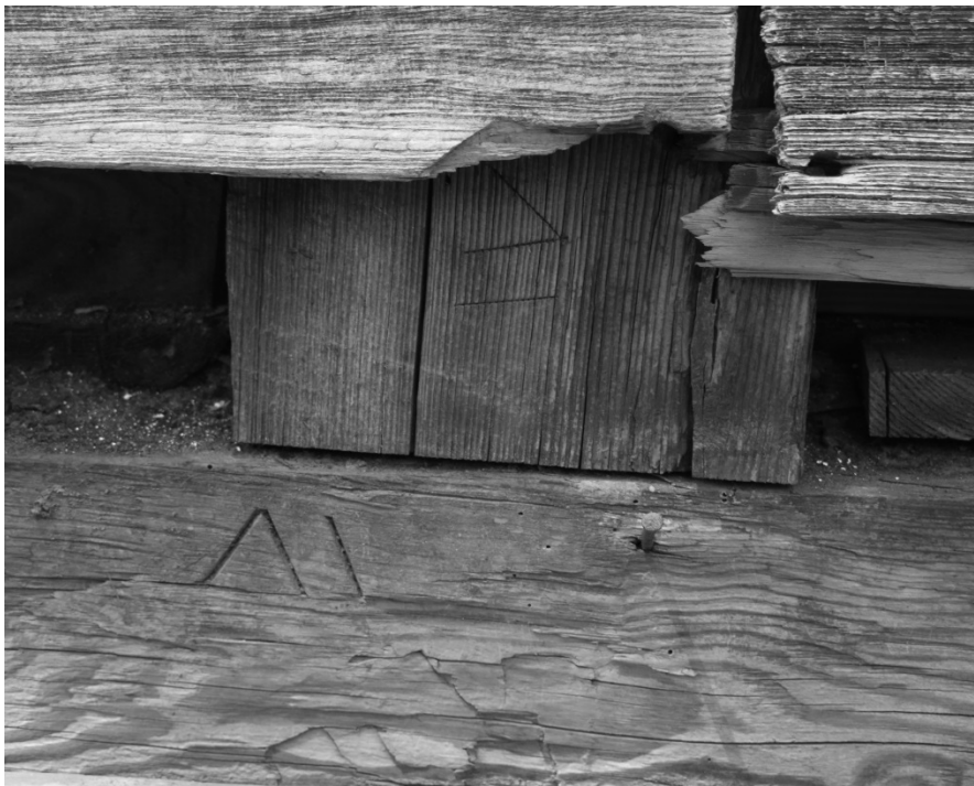
Figure 8: carpenter’s numeral on matching timbers
