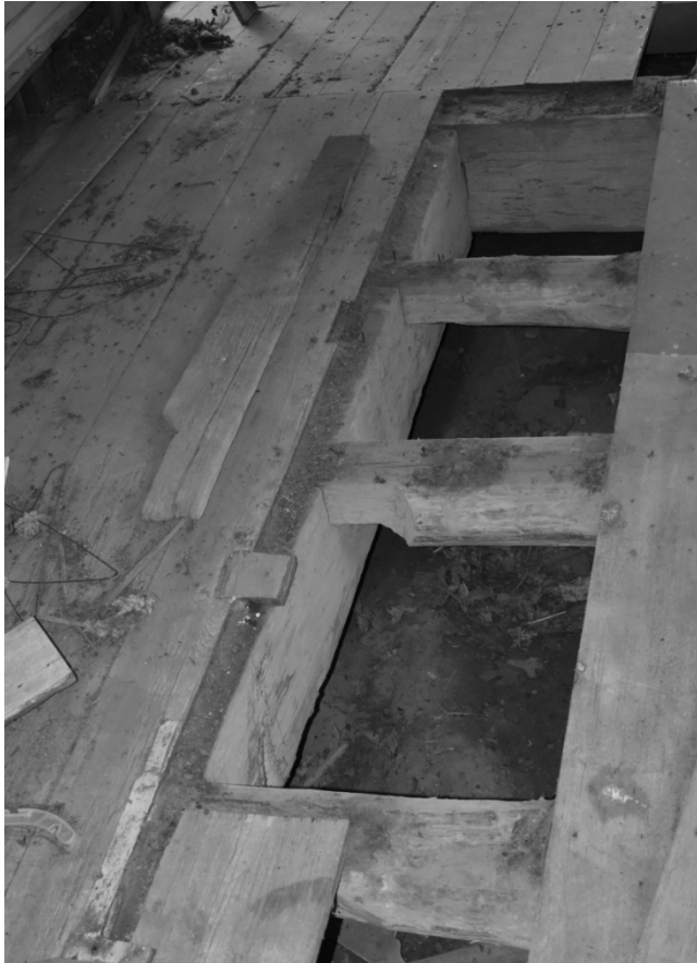
Figure 5: typical floor joists seen from above
