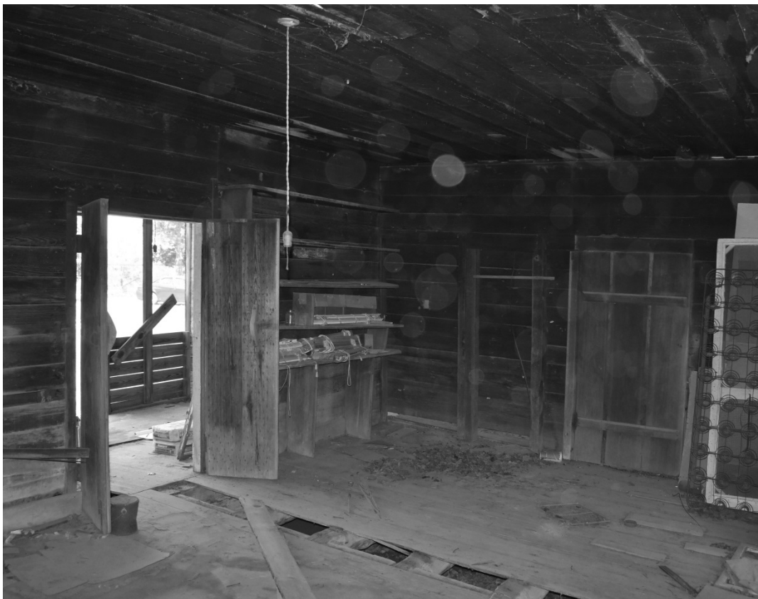
Figure 21: Room 101, looking northeast
