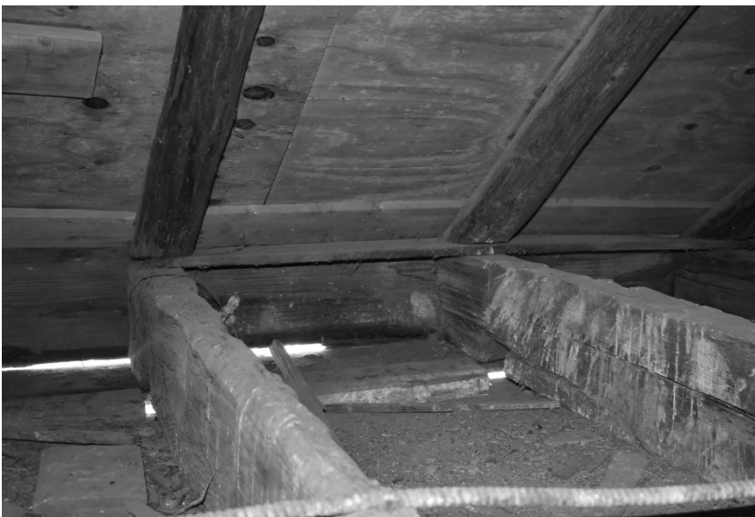
Figure 11: Ceiling joists, false plate, and rafters in attic
