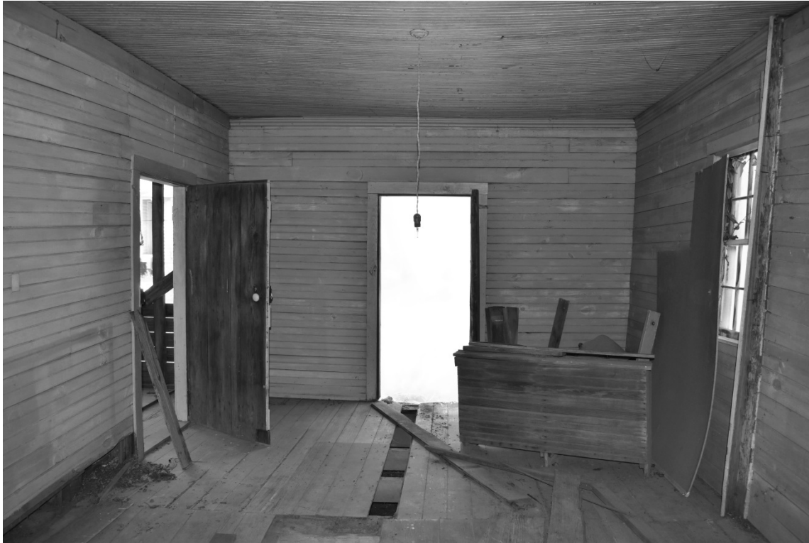
Figure 27: Room 104, looking north
