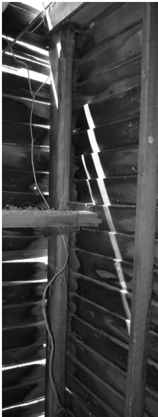
Figure 23: original porch post in northwest corner of Room 102
