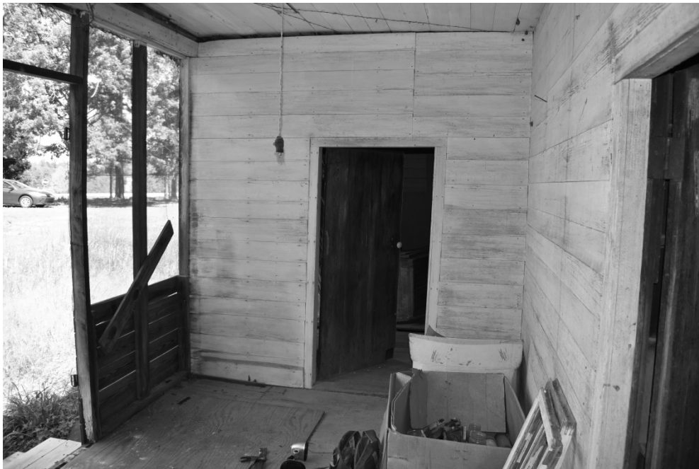
Figure 25: Room 103, looking east
