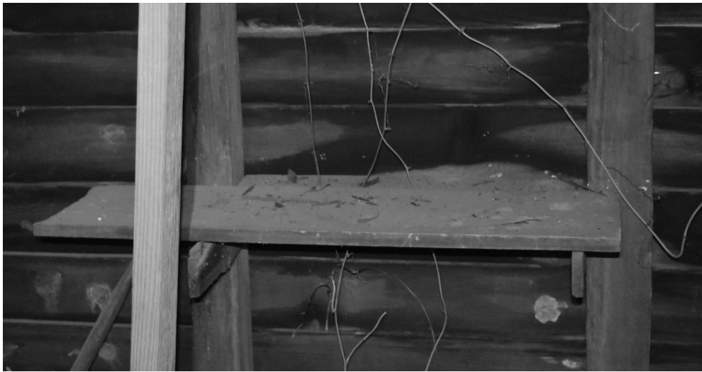
Figure 16: Shelf in attic
