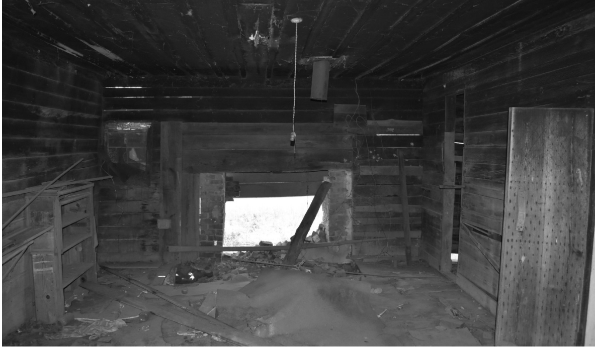
Figure 18: Room 101, Kitchen, looking west towards fireplace
