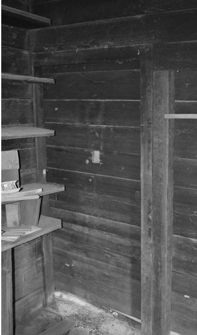
Figure 19: Room 101, former door frame in NE corner to quarters
