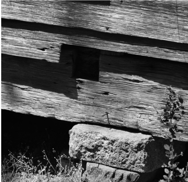
Figure 6: mortise in sill for former rear porch
