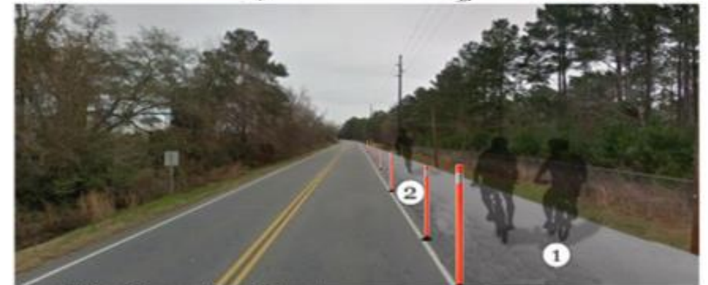
Paved Shoulder on S. 3rd Street
