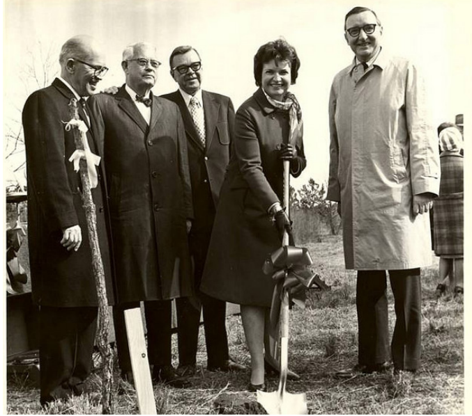
The first groundbreaking of EGSC's campus.
