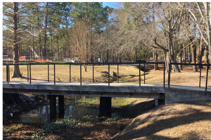
Bridge across Ezra Pond.
