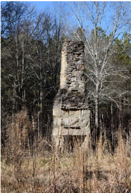
Figure 11 (Page 41): Remaining chimney at Hilton Homeplace, circa 1870s
