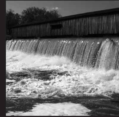
Watson Mill Bridge, October 2009
