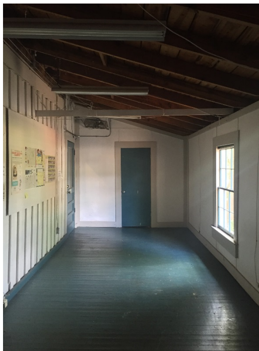
Exterior of same gym wall on left, as seen from porch (visibly bowing outward)
