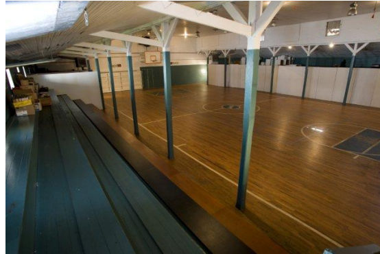
Interior view of court from N corner
