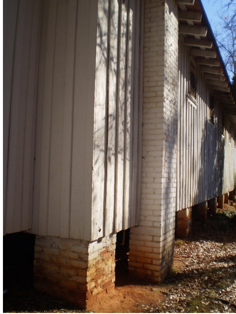
Red clay backsplash on brick piers and southwest chimney
