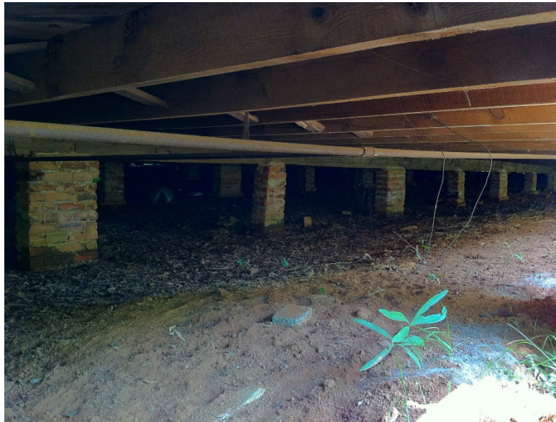
Brick piers beneath the gym, as seen from the southwest side
