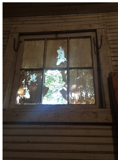
SW "Visiting Team" locker room window, paned
