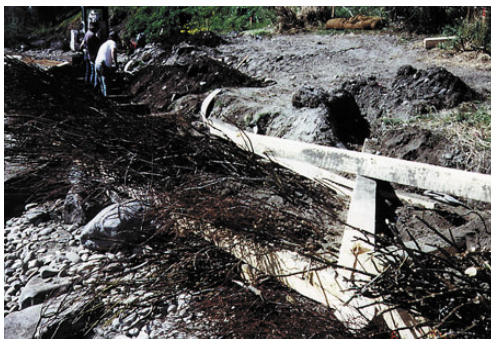
Vegetated cribbing under construction
