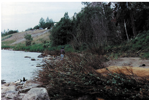
Vegetated cribbing post construction
