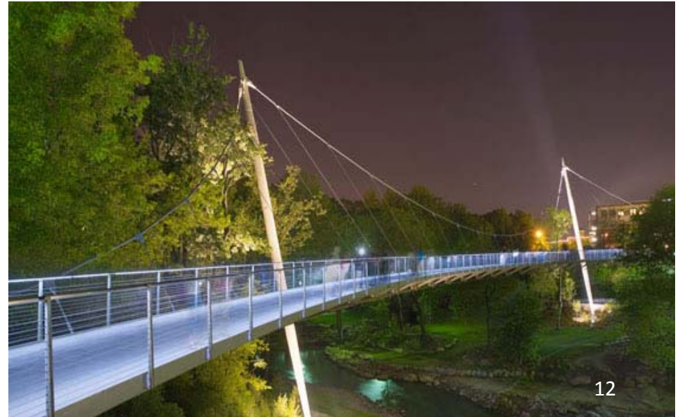
Example: Suspension Bridge (Falls Park, Greenville SC)
