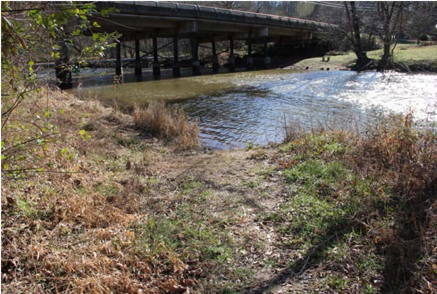
See the natural eddy formed by the inside bend of the river, which is created by a natural gravel bar upstream held by River Birch trees.
