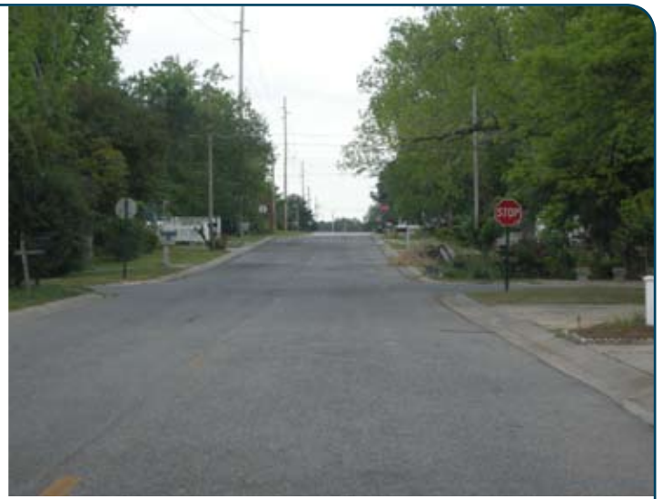
This photo from the Westside neighborhood directly across 16th Avenue illustrates the stormwater solution practiced throughout Cordele.
