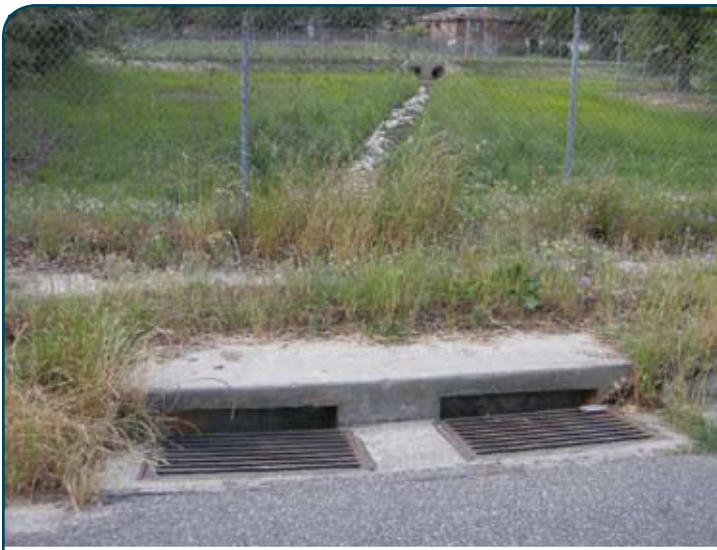
This drainage field in the Westside Neeighborhood.
