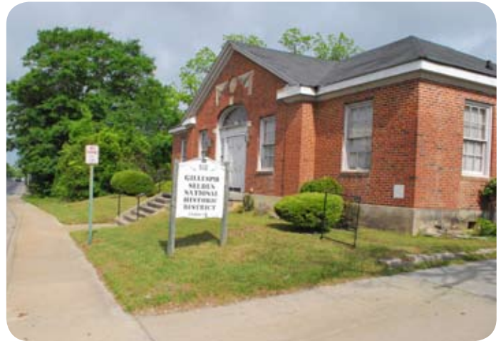
The hospital is in good condition but the longer it remains vacant, the more potential for deterioration.
