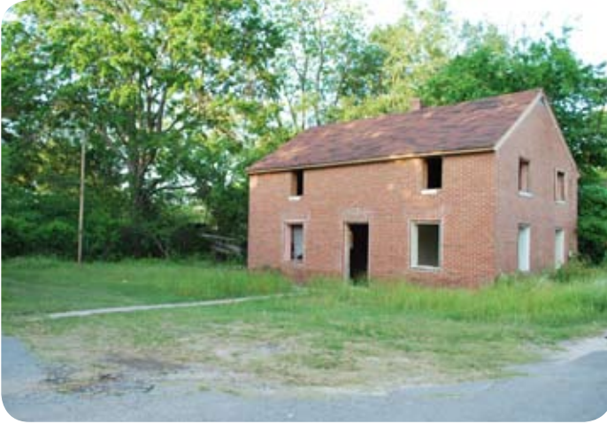
This is the current condition of the Nursing Quarters Building.
