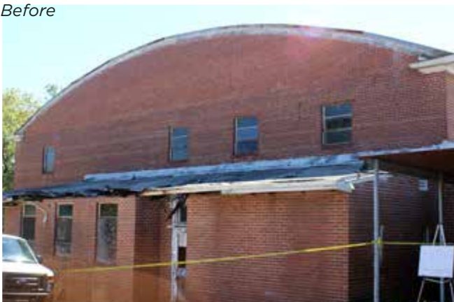
The shed-roof storage rooms can easily be removed from the building to allow for the introduction of a larger opening to accommodate indoor/outdoor events.
