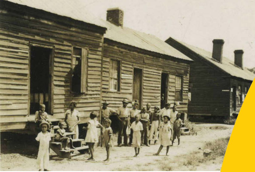
Nineteenth-Century View of a Rural African American Small Village or Hamlet, Augusta-Richmond County Area. The early Springfield landscape probably resembled this kind of loosely organized village or hamlet containing a few buildings surrounded by much vacant land. (Source: Augusta Museum of History).
