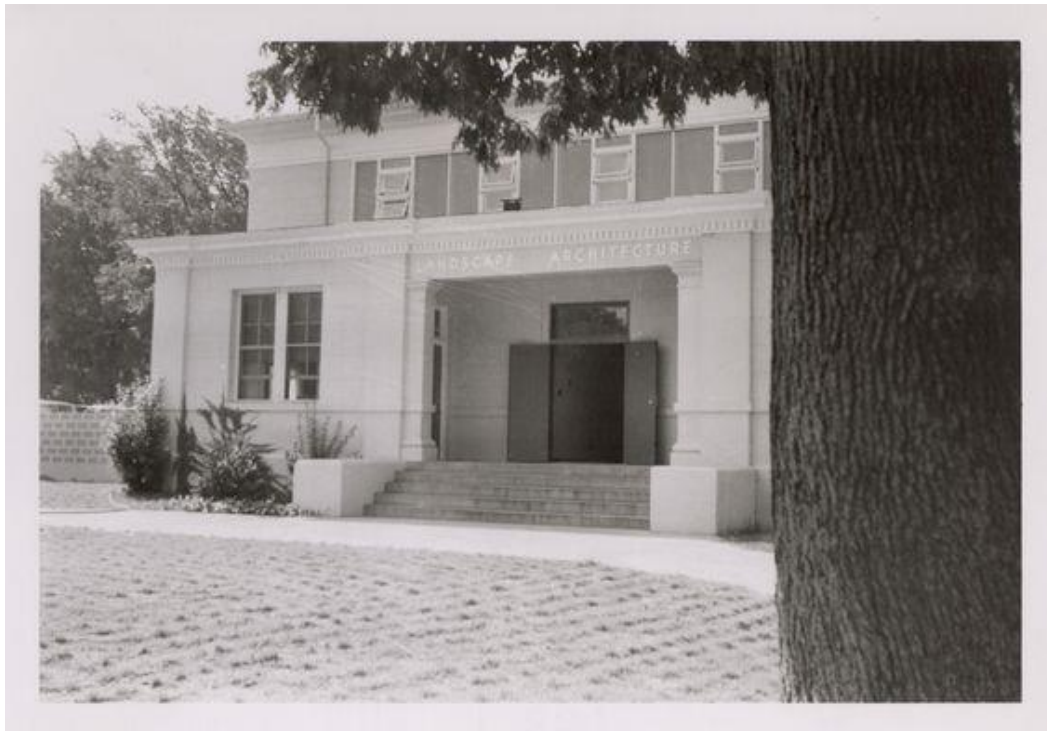
Fig. 1.5: Photographer unknown. North façade of Denmark Hall as the Landscape Architecture Building.
